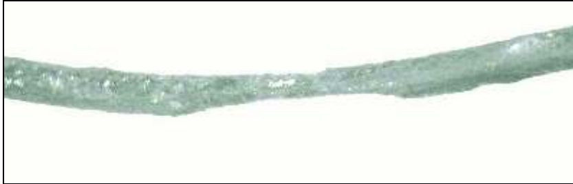
Figure 11. Outer wire of outer strand showing abrasion at the contact points as well as corrosion.
